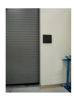
The MR-1824's attractive enclosure comes in dark gray. Its electronics and antenna are potted in UL-approved epoxy resin potting compound to seal them against adverse environmental conditions. It is manufactured in an ISO 9000 certified facility providing for the highest quality standard.
